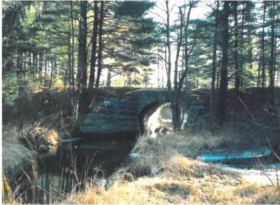
1989 view of Arch Bridge from Flat Rock Quarry property
